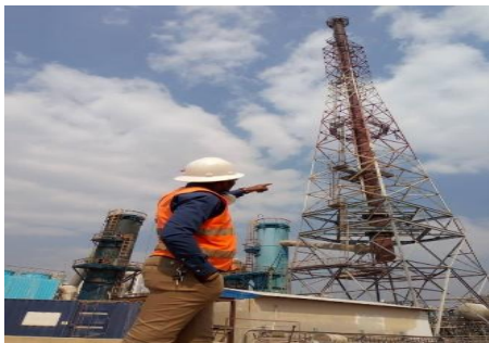
Figure 14 : Sulfuric acid plant chimney (shutdown due to Annual Shutdown)
